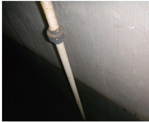
Most pipe lines that go from close to the bottom of the cistern to the pump have a filter on the end, these filters may become clogged over time. A good reason to keep your gutters and gutter screens clear to limit the amount of debris getting into the cistern. The fine sediment at the bottom of the cistern is Sahara dust that rain picks up as it falls, or washes from the roof.
