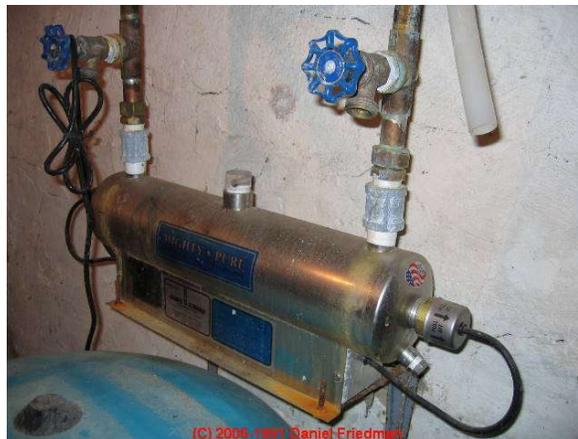
UV dis-infection is very quickly gaining ground on other conventional disinfection processes because it is effective, environmentally friendly and economical. UV does not change the taste of water and does not add anything to it. For many applications, it is the ideal choice for disinfecting water.
