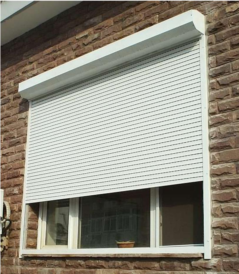
Roll down can be manual or powered. Be sure to have the manual key should the power fail.
